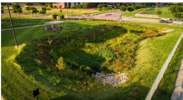
Detention Pond Amenity at Entrance
