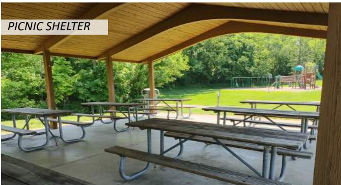
15 The painted metal drip edge is warped at some locations, as are the wood rakeboards
