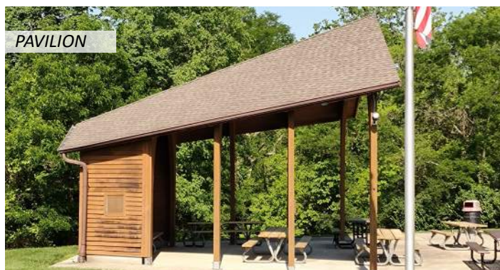
23 The asphalt shingle roof, gutter and drip edge appear to be in good condition
