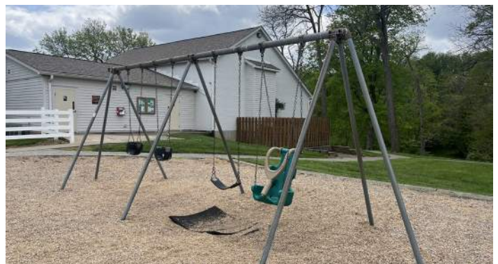
6 Swings appear aged and concrete edge of playground is heaving in areas
