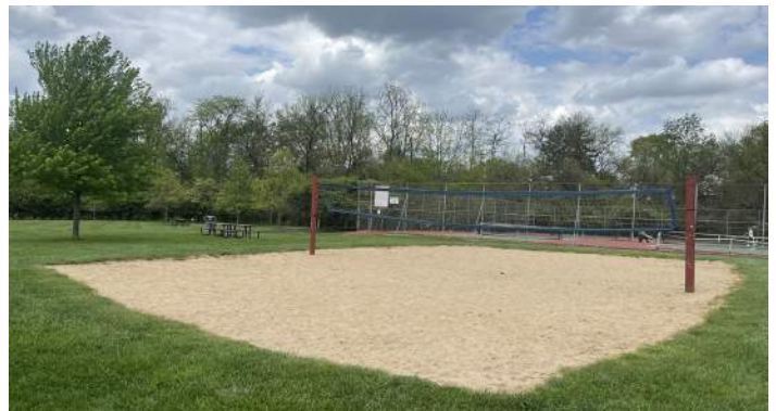
4 Sand volleyball net and poles in poor condition with no barrier between sand and grass
