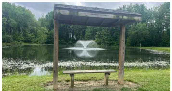
30 Benches with overhead cover are weathered and appear to have moisture damage to the roof
