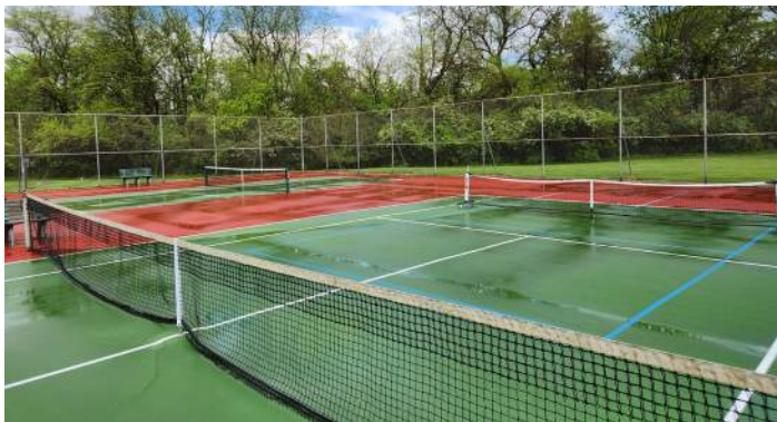
3 Tennis nets and posts appear to be in poor condition but minor cracking appears on surface
