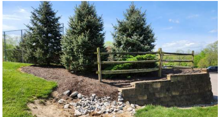
14 Landscaping appears to be washed out in sloped areas and decorative fence is weathering
