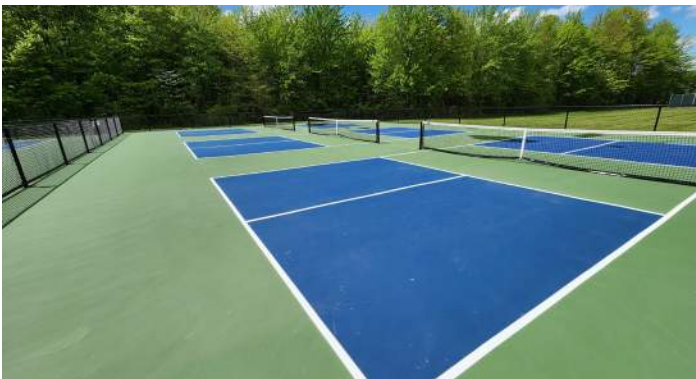
3 Newly constructed pickleball courts are in good condition
