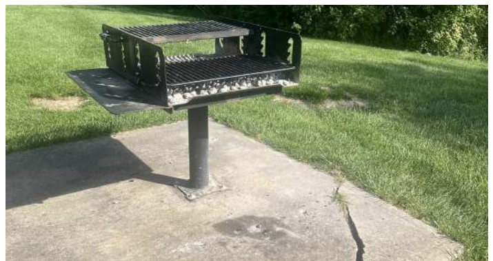
12 Charcoal grill is in fair condition, with its concrete pad needing repair
