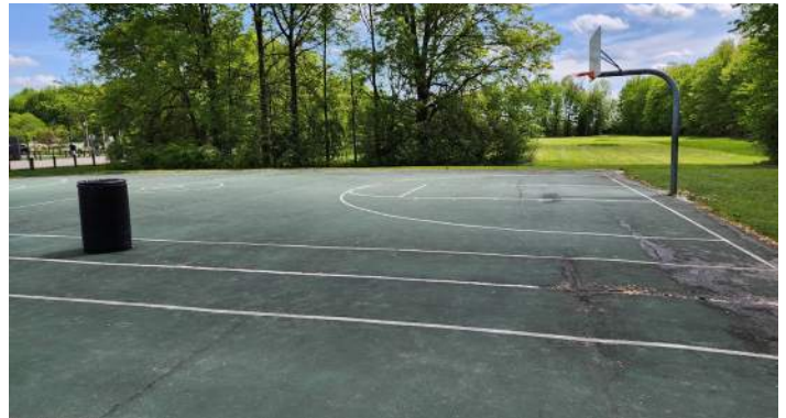
2 Basketball surfacing is cracking, discolored, and in need of repair
