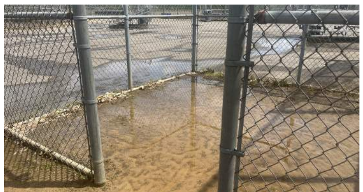
6 Infields appear to be sloped toward the dugouts and backstops, causing significant wash out
