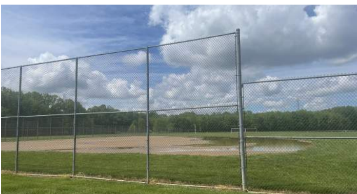
5 Infields present many drainage issues and ponding while outfields tend to drain better
