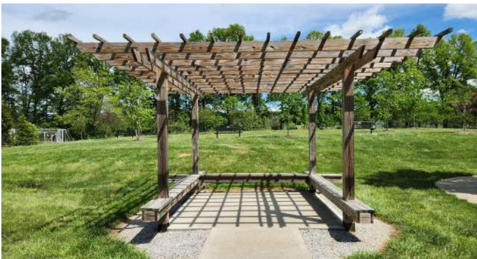
27 Seating area with overhead pergola appears in good condition
