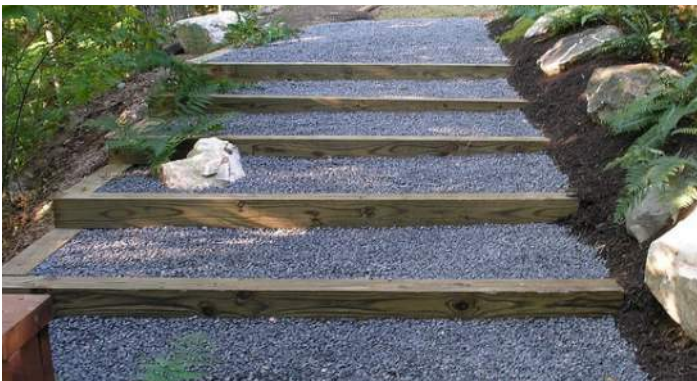
Updated staircase with gravel treads and slip-proof risers
