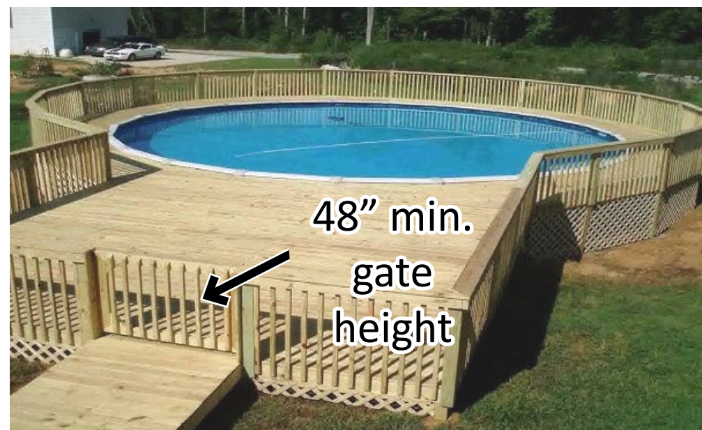
On a deck around an above ground pool, the fence and gate shall be at least 48" tall. A self-closing, self-latching gate is required.
