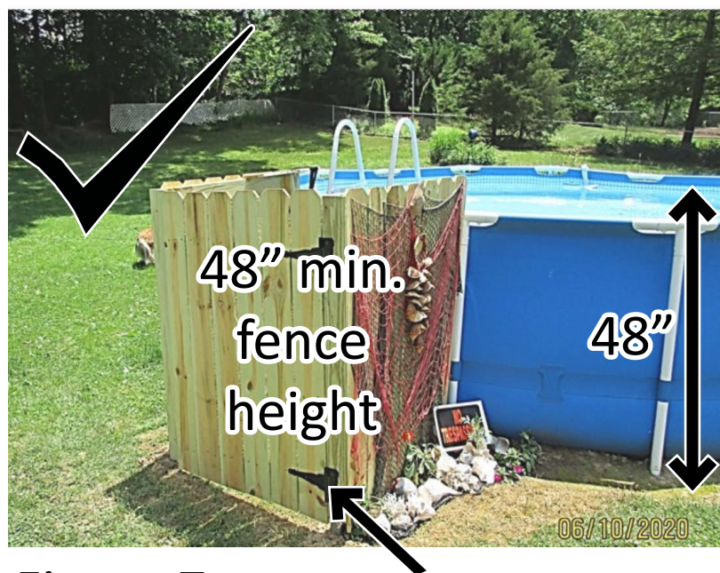
Figure 7 Mount gate high enough to not drag on the ground!
